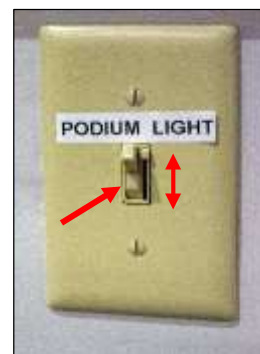
Podium Light Switch (on/off & dimming slider)
